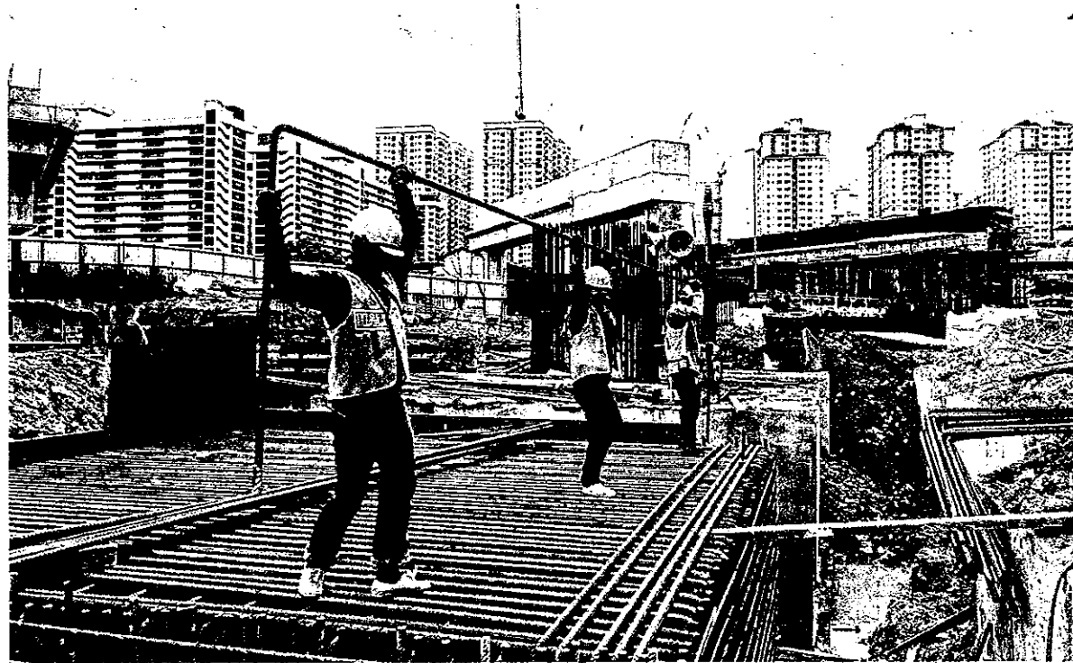
Good prospects: Maybank IB says construction companies with healthy order books will benefit the most as infrastructure projects pick up. — Bloomberg
